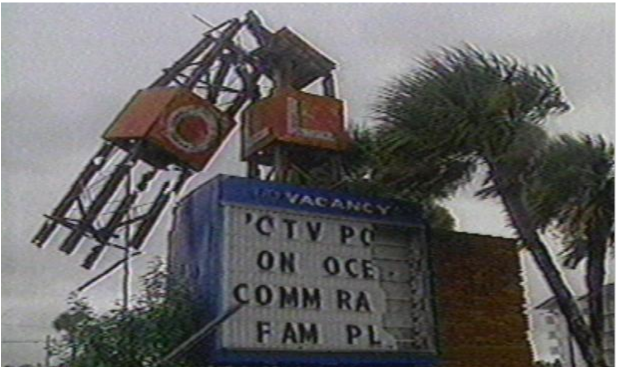
Hotel sign blown down
