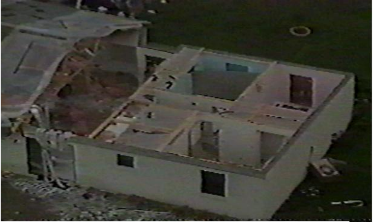
Tornado removes roof from house east of Orlando.
