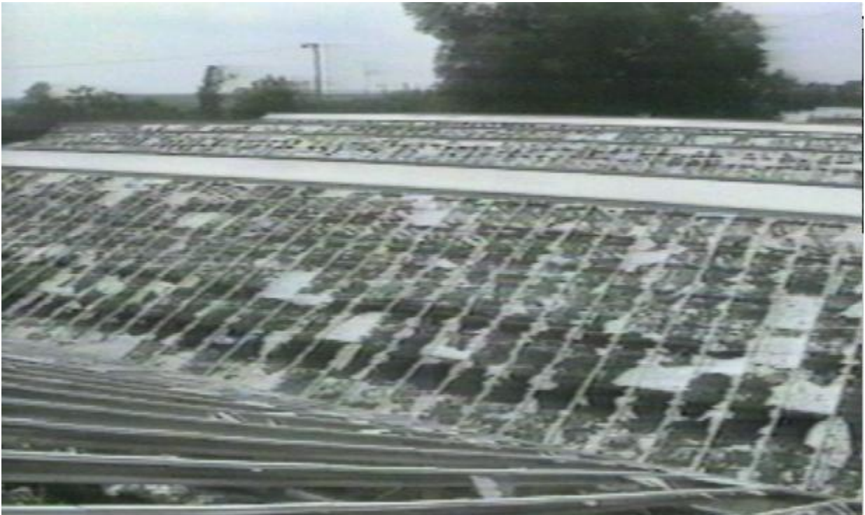
Widespread greenhouse damage from large hail.
