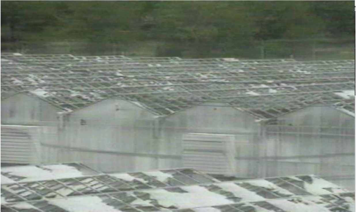
Widespread greenhouse damage from large hail.
