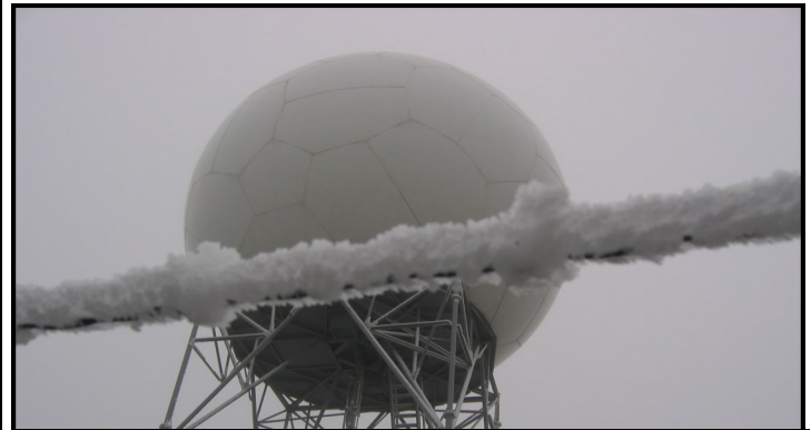
Rimming on the fence near the NWS Spokane radar on 1/23/14
