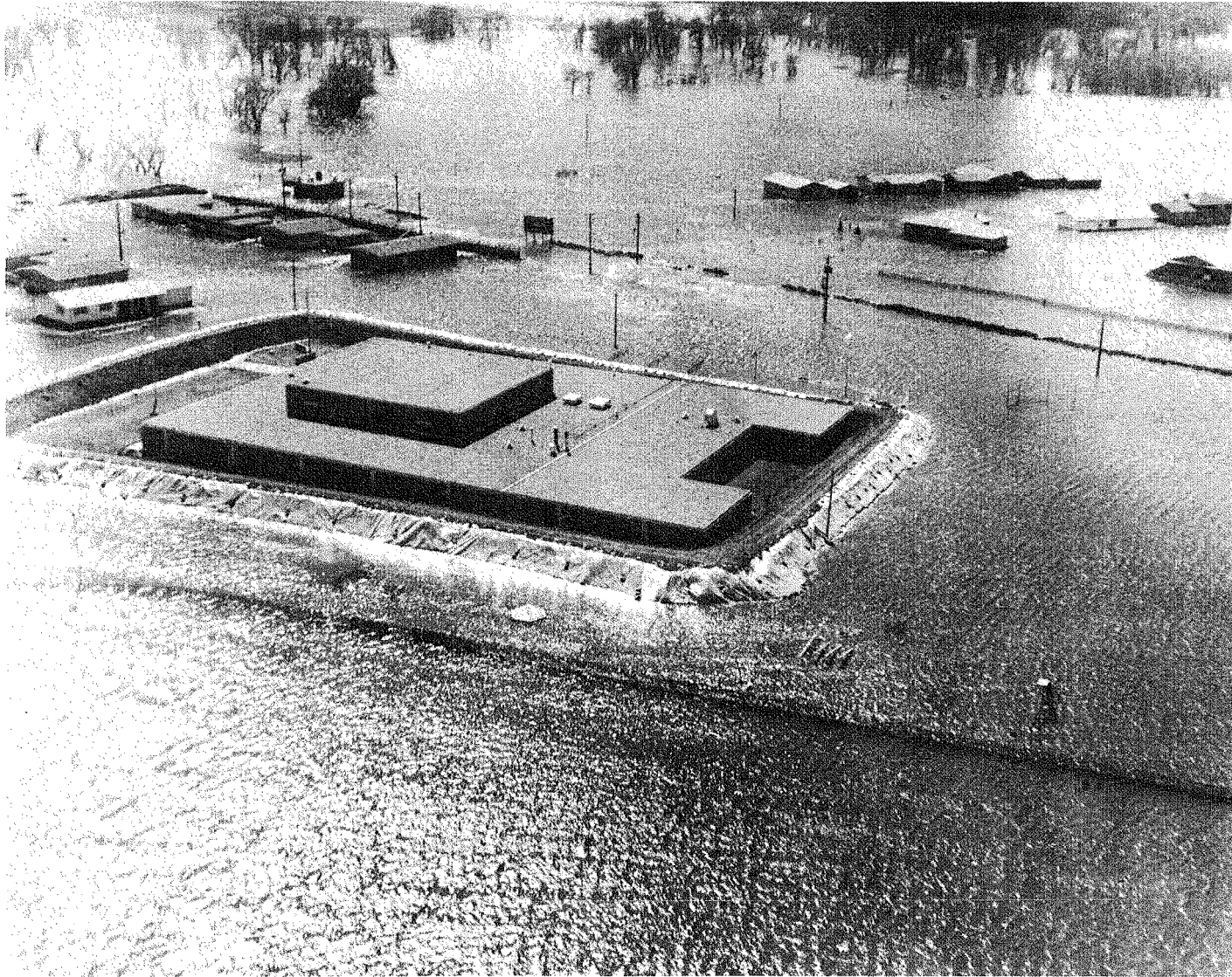
School in Minot, N. Dak., protected from flood waters by emergency dikes erected on basis of early warnings. Photographed by North Dakota National Guard on April 11, 1969, 8 days before flood crested.
