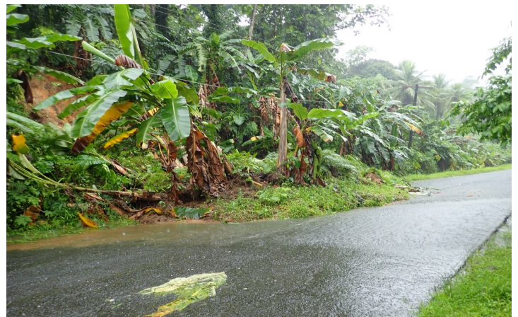
Landslides covering half the road at Madolenihmw
