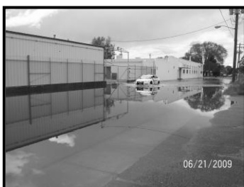
Blackfoot Flash Flood 2009
