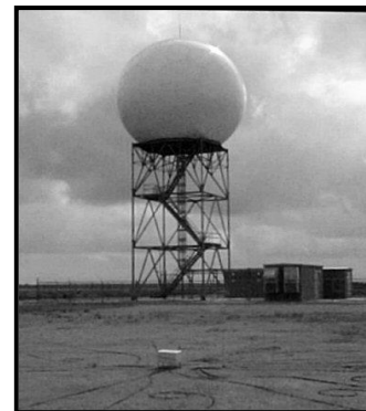
NWS RADAR RADOME
