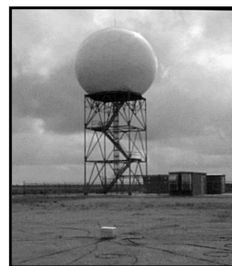
NWS RADAR RADOME
