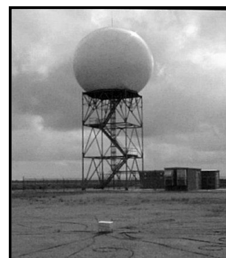
NWS RADAR RADOME
