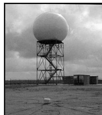
NWS RADAR RADOME
