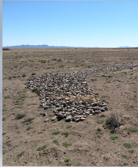
Channel Restoration Area
