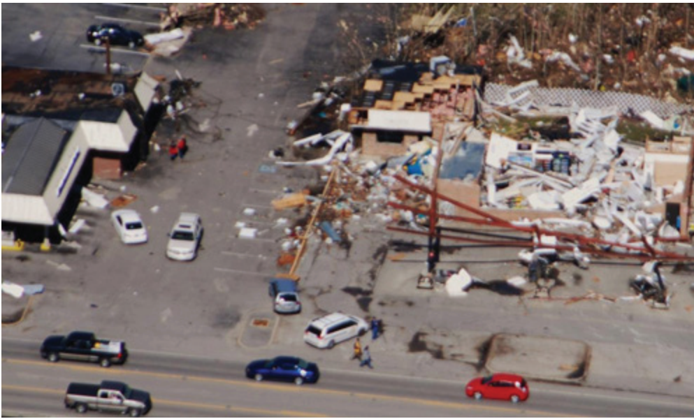
Shown at right are the remains of the Mighty Mart grocery store after a tornado tore through Saylorsville, KY. Thanks to a warning by StormReady Hero Doc Hardin, staff and customers sheltered in the cooler room minutes before the tornado struck. The room was the only part of the store not destroyed by the EF-3 tornado.
