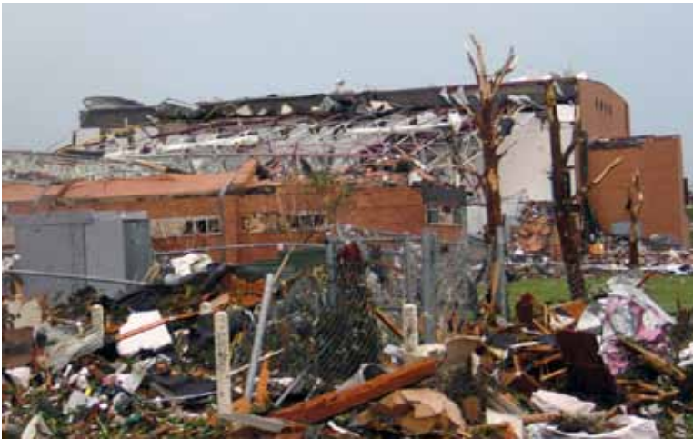
Devastation caused by Joplin, MO, Tornado, May 22, 2011
