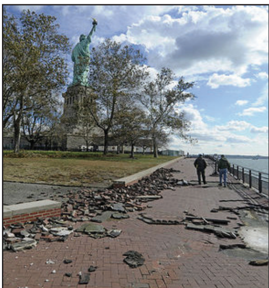
Brick pavers dislodged from Sandy's storm surge. From Flickr, SandyResponseNPS
