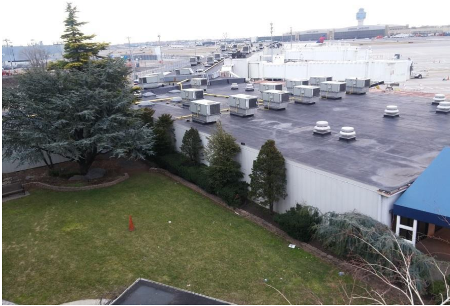
Looking east from the roof of the Marine Air Terminal toward the primary snow measuring area at LaGuardia Airport. The orange cone is the location used for measuring snow.
