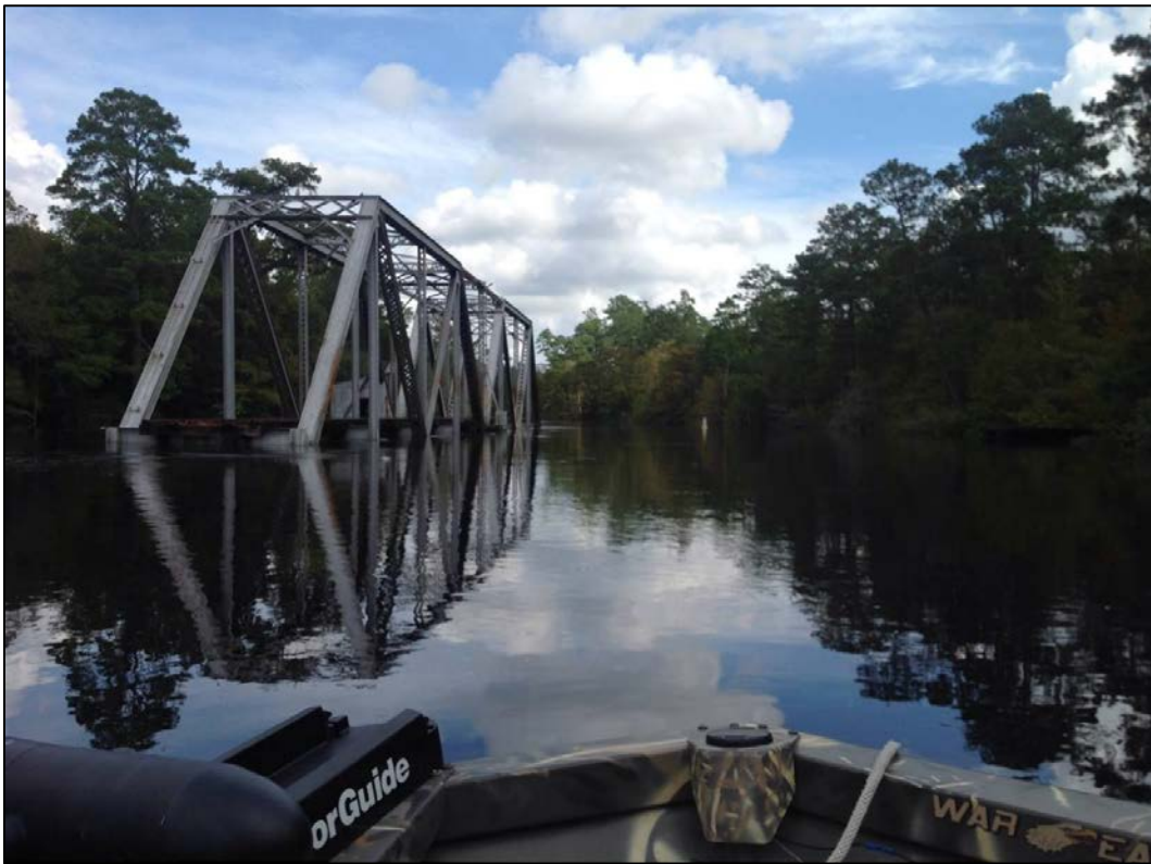
Figure 13: Waccamaw River Floods out Railroad Bridge Flooded in Conway, SC. Source: USGS
