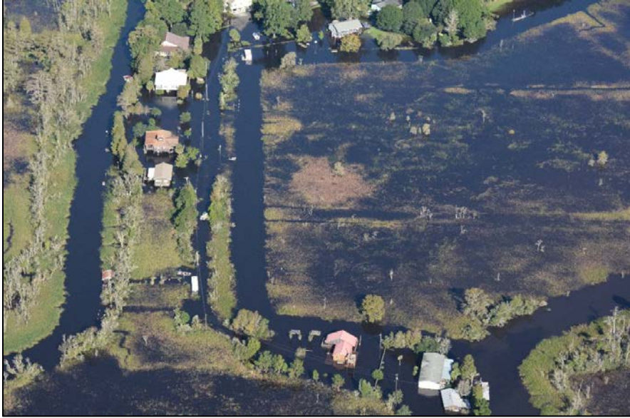
Figure 12: Flooded homes in Georgetown, SC. Source: USGS
