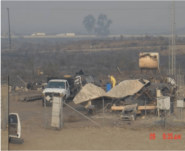
Picture 2. Destroyed office and storage trailers at Upper Air Facility. Courtesy of WFO San Diego.
