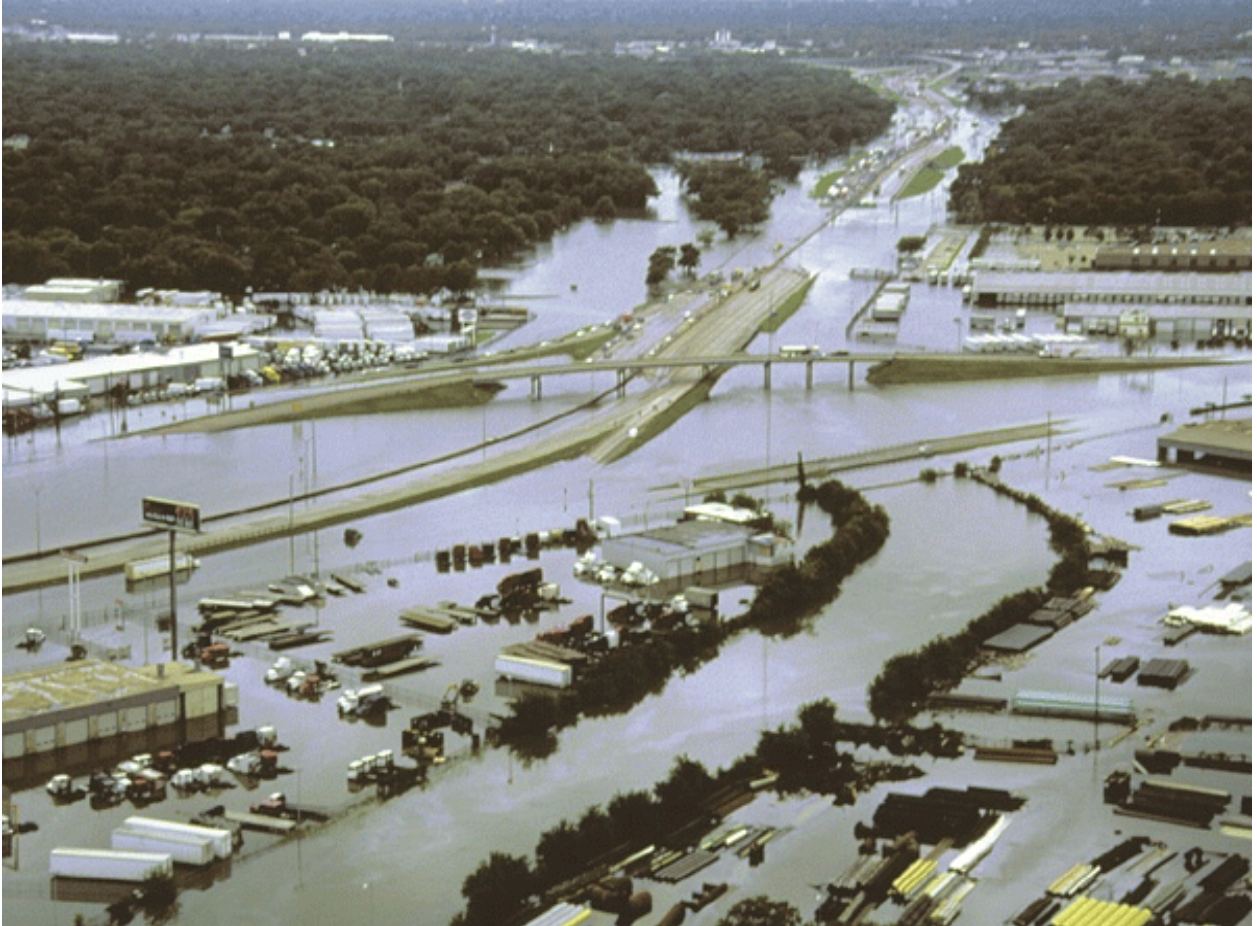
Interstate 10 North Loop, Houston, Texas. (Courtesy of Harris County Flood Control District/ Steve Fitzgerald)
