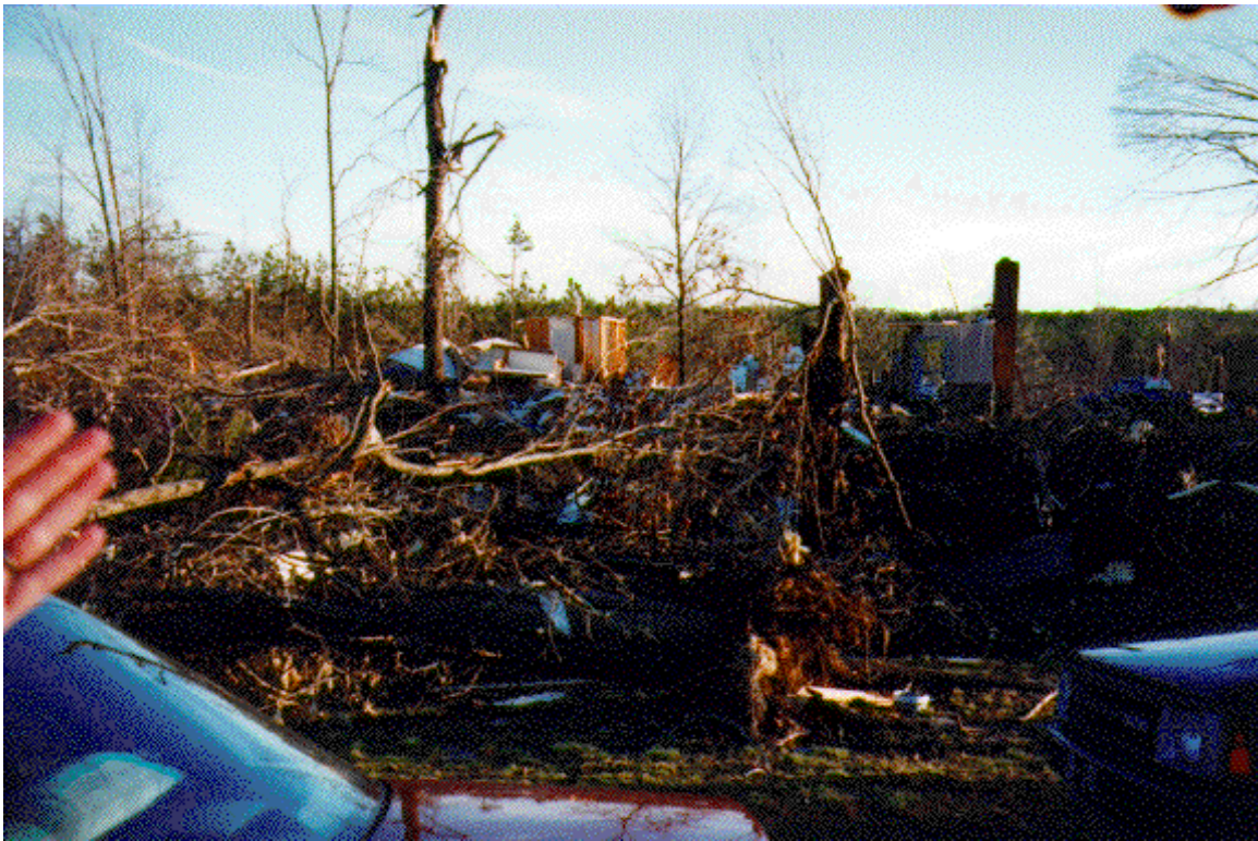
This photograph shows the tornado damage in the Vimy Ridge area of Saline County. All of the homes were damaged and nearly all of the mobile homes and frame houses were destroyed. Pictured is a destroyed home with only a chimney and parts of two walls remaining. Courtesy of Chris Smith, NWS Southern Region.
