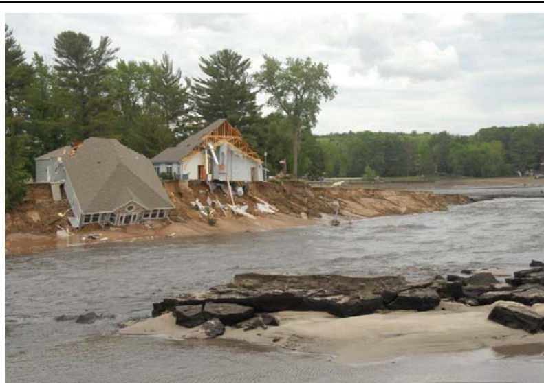
Fig. 14. Homes were destroyed on Lake Delton in Wisconsin when the 245-acre lake quickly emptied after Dell Creek cut a new channel into the Wisconsin River, bypassing the dam. (U.S. Air Force photograph by Master Sergeant Paul Gorman.)
