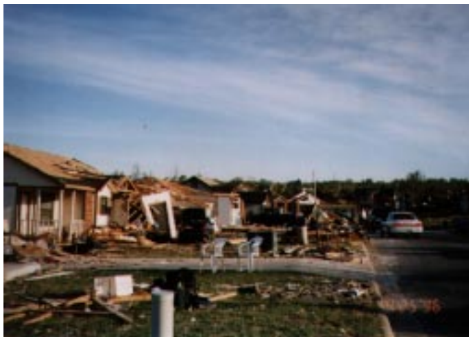
F3 Damage, Vista Ridge subdivision, Van Buren
