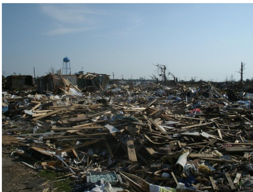
Figure 14: Damage in Smithville, MS (courtesy of WCM Chance Hayes, Wichita, KS)
