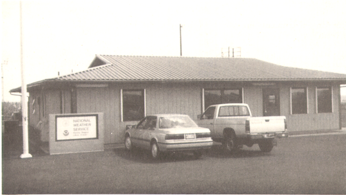
Figure 2. WSO Lihue Following Hurricane Iniki (Photograph Courtesy of William Alder)
