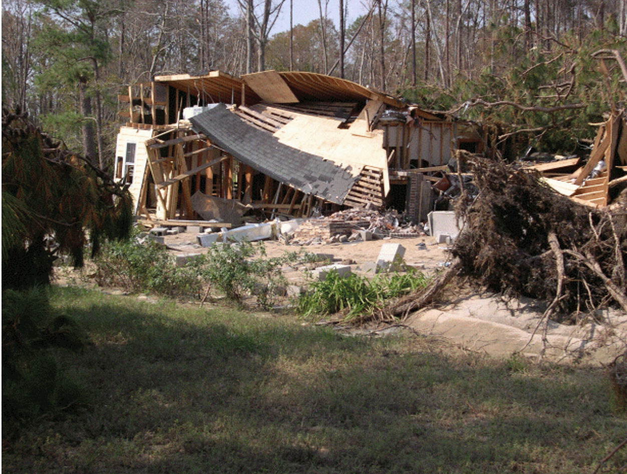
Picture 2. A small cluster of four homes about 5 miles west of Edenton, NC, occupied year-round were completely destroyed by the surge, two of which were moved up to 20 feet off their concrete block foundations. (NWS Isabel Assessment Team photo by Dave Vallee.)
