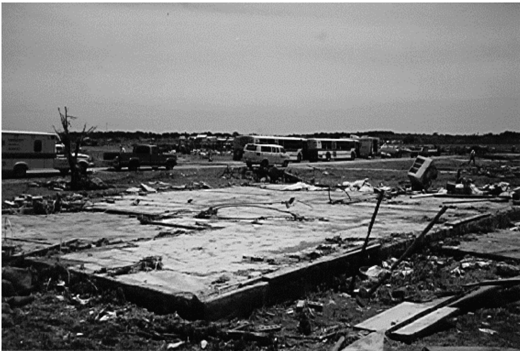
Close-up view of a home foundation in the Double Creek Estates subdivision of Jarrell. Note the plumbing pulled out of the concrete in the center of the picture. Photograph by NWSFO Austin/San Antonio.
