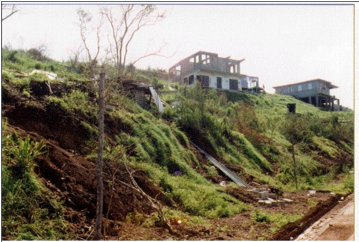
Figure 1-17. Homes destroyed on Culebra by Marilyn. (Photo courtesy of Kevin McCarthy)
