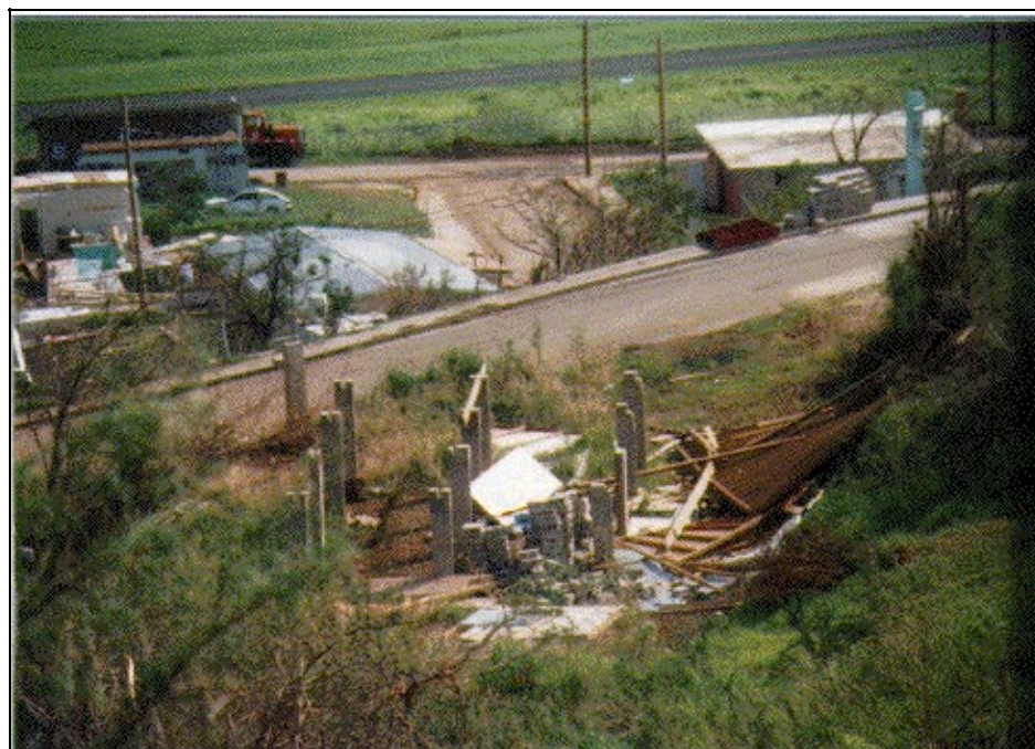
Figure 1-19. Home flipped off its pilings. (Photo courtesy of Reggina Garza)
