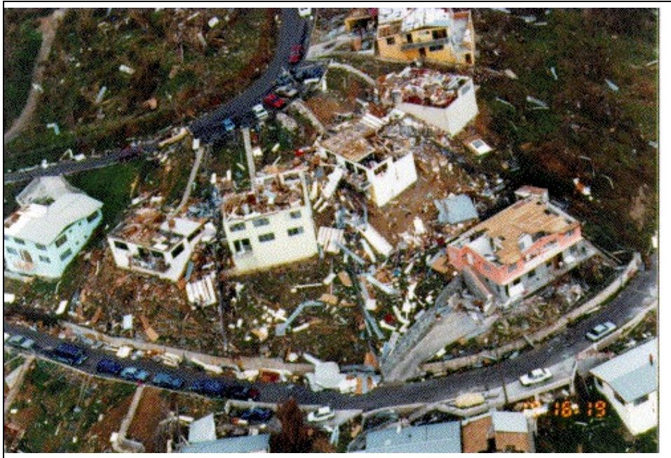
Figure 1-15. More damaged homes on St. Thomas. (Photo courtesy of Brian Smith)
