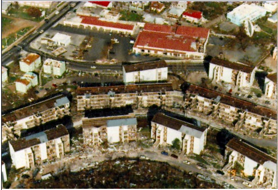
Figure 1-11. Destroyed apartments in Charlotte Amalie. (Photo courtesy of Brian Smith)
