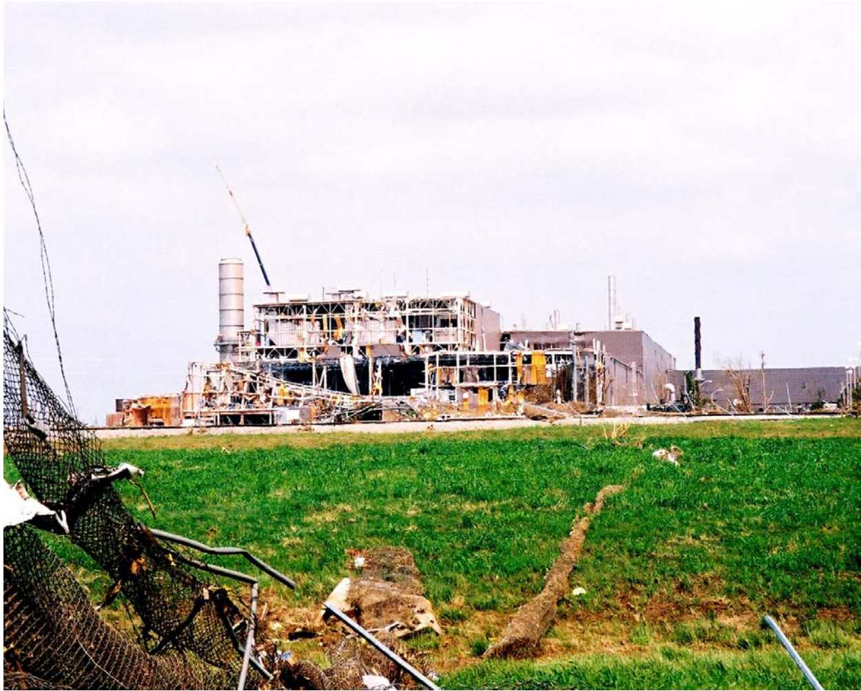
The General Motors Manufacturing Plant in southeast Oklahoma City after the May 8 tornado.
