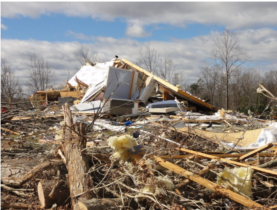
Fig. 7c. Damage to a home in the Evergreen area.
