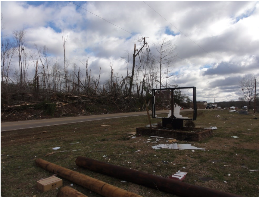
Fig. 4a. Damage along Ararat Highway.
