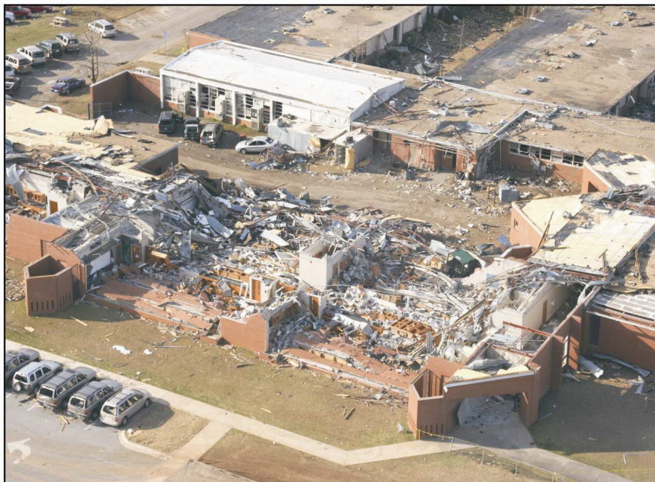
Figure 5. Significant destruction at Enterprise High School where eight were killed.
