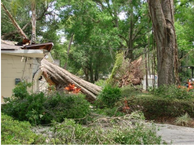
Uprooted tree that fell on a house on Grand Circle
