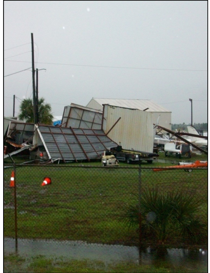
Tornado at Position 4 : Power poles and lines snapped with numerous trees down in area. Downburst wind at Position 5 : Damage to a small metal hanger at the St Pete/Clearwater International Airport with wind estimated at 60 MPH. The weather instrument on other side of airport recorded 55 MPH winds at 11:21 AM. A tractor trailer overturned on the Interstate 275 at Position 6 .
