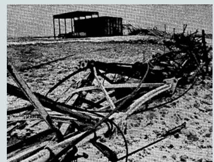
Figure 3 Twisted skeleton of the 1439 foot tower of KLDH-TV in Topeka, KS. The tower buckled and collapsed under the weight of a 3 inch thick coating of ice. -Photo by Kathy Borchers, Topeka Capital-Journal
