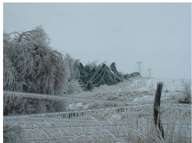
Heavy ice accumulation was incredibly detrimental to the structural integrity of trees and power lines.
