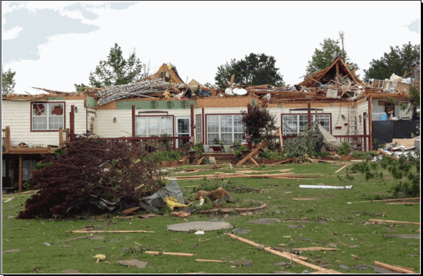
An EF2 tornado severely damaged a house in Broken Arrow in Wagoner County, Oklahoma, during the evening of May 30, 2013. Photo by Ed Calianese, WCM, WFO Tulsa.
