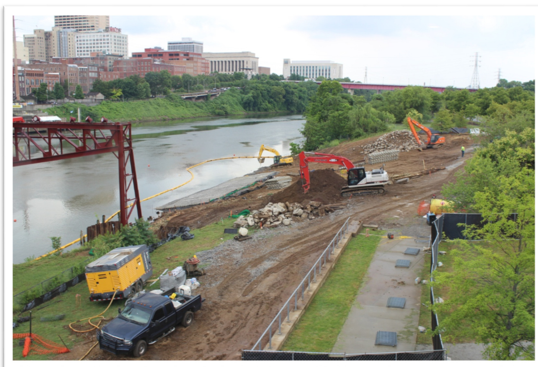
Boat ramp construction, Cumberland River, Nashville, Tennessee. Photo: Bob Sneed, USACE
