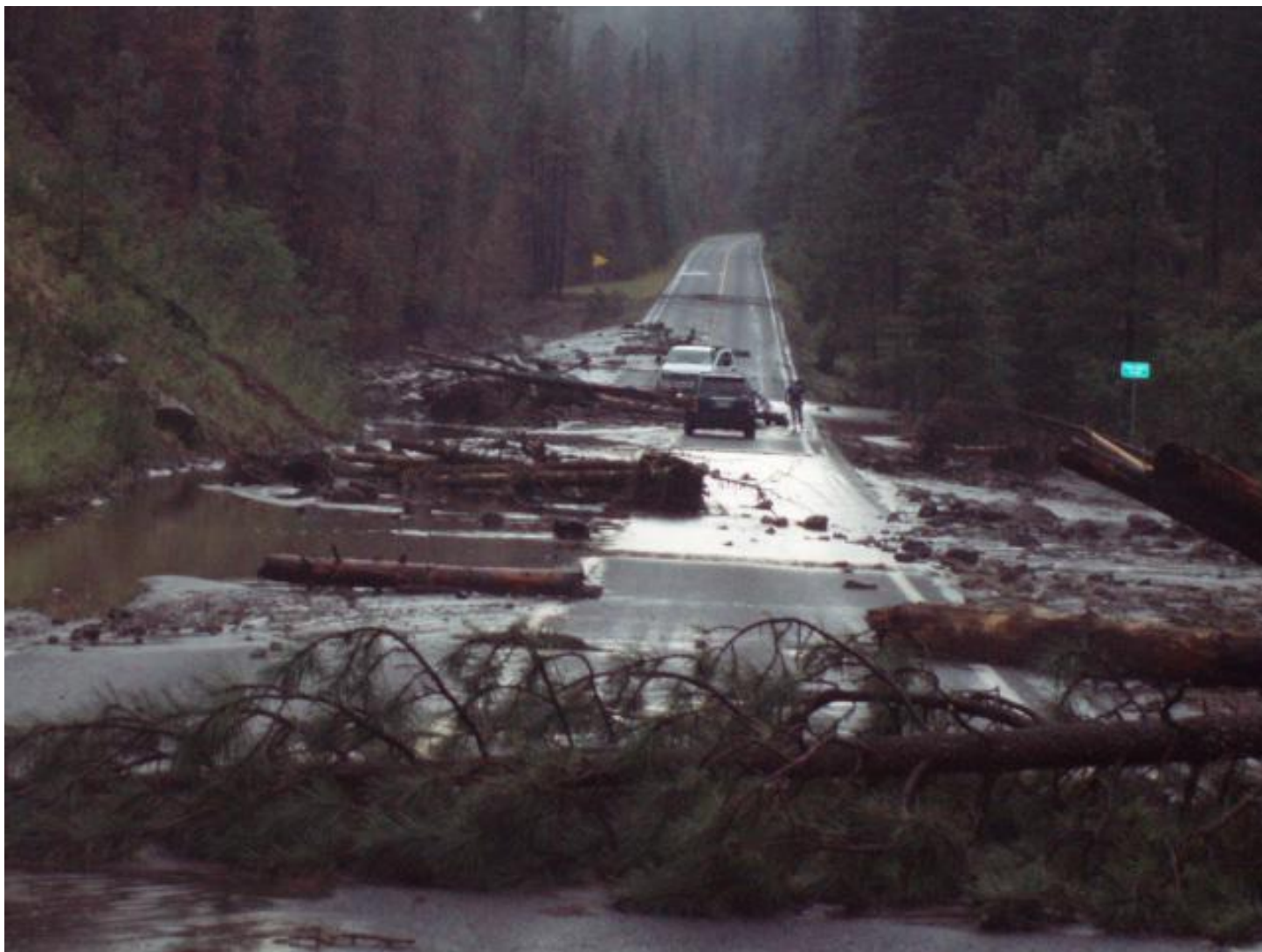
Figure 79. Hannagan Creek Basin at Highway 191 (photo provided by AZDOT). Culvert became blocked and Hannagan Creek flowed over Highway 191. Flow was 4-8 feet deep over road above culvert (near where person is standing in photo). Perpendicular to direction of flow, from highwater mark to highwater mark, was a distance of 980 feet (in photo you can see far highwater mark near yellow sign). The highwater marks were likely not made at the same time. Also, the flow across the road may have at times been braided or the direction of flow may have not always been perpendicular to the road. Cross Section #2; Main watercourse over road estimated as 30 feet wide, 6 feet deep, having a shape of half an ellipse, a wetted perimeter of 36 feet, a n value of 0.055, and a slope of 0.022. Estimated flow = 1,405 cfs. Mean velocity = 10 ft/sec. [Estimated flow = 1,360 cfs using a broad crested weir equation 24 with hydraulic head (H) = 6 feet, weir length (L) = 30 feet, and discharge coefficient (C) = 3.09.]
