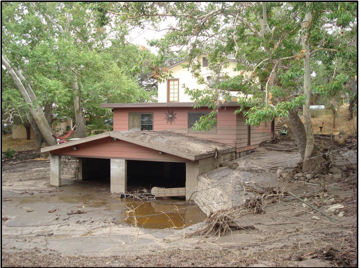
Figure 18. Notice the debris on the car port roof and highwater mark stain on the two shown sides of the building. This photo was provided courtesy of BAER team and was taken the day after the lower Miller Canyon flash flood.
