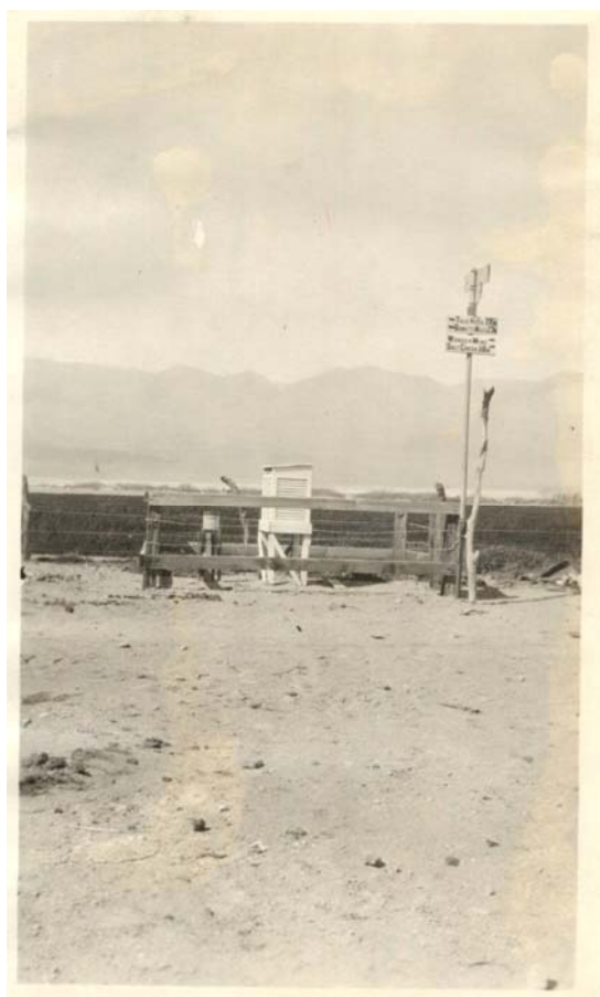
This picture of the weather station at Greenland Ranch in Death Valley was taken during a station visit in March 1924 prior to the rain gauge being moved. Photo Credit: NWS Las Vegas archives.
