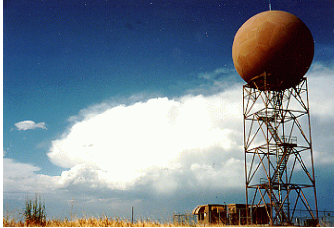
Figure 45. Boise's WSR-88D Doppler Radar (KCBX). Date: Unknown. Source: National Weather Service Boise, Idaho Archives.
