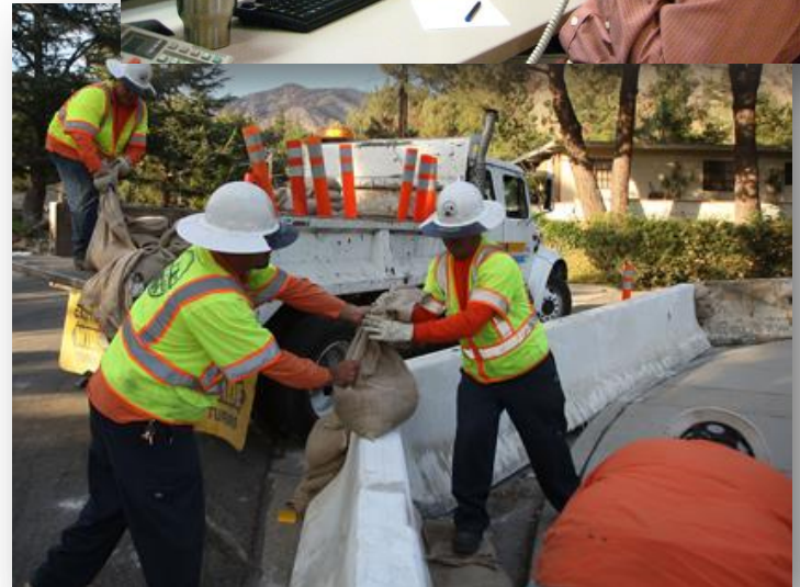
Los Angeles County Public Works deploying K-Rails below burn area prior to expected heavy rains (Photo credit: Getty Images)
