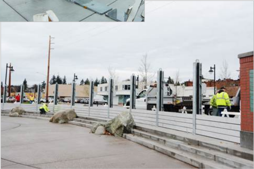
Mount Vernon flood wall
