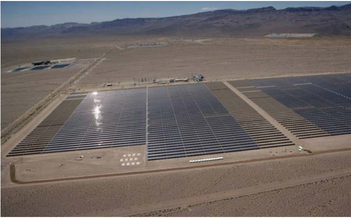
Figure 5: 64 MW Nevada Solar 1 Solar Plant
