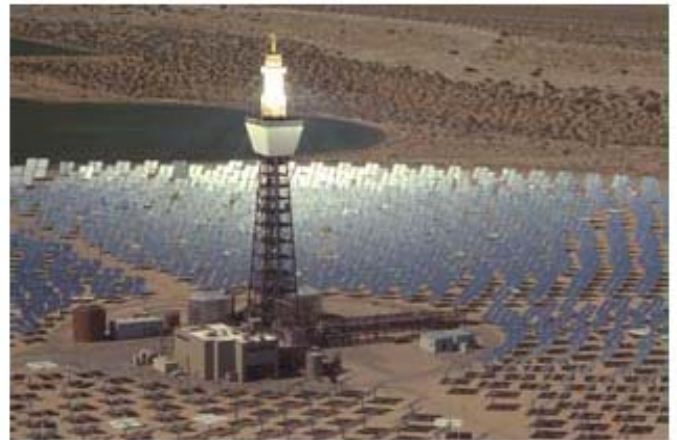
Figure 8: 10 MW power tower pilot project, Barstow, CA
