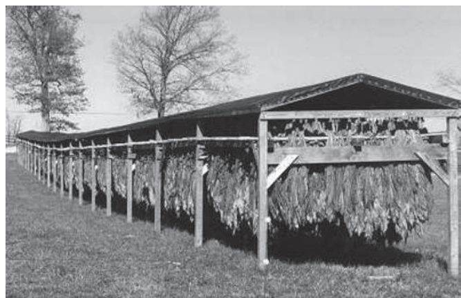
A gable-roof structure.
