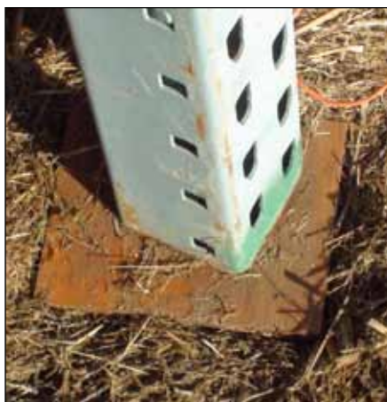
Figure 11. Wooden pads, approximately 6 inches x 6 inches, placed under pallet rack uprights that lack attached metal pads.
