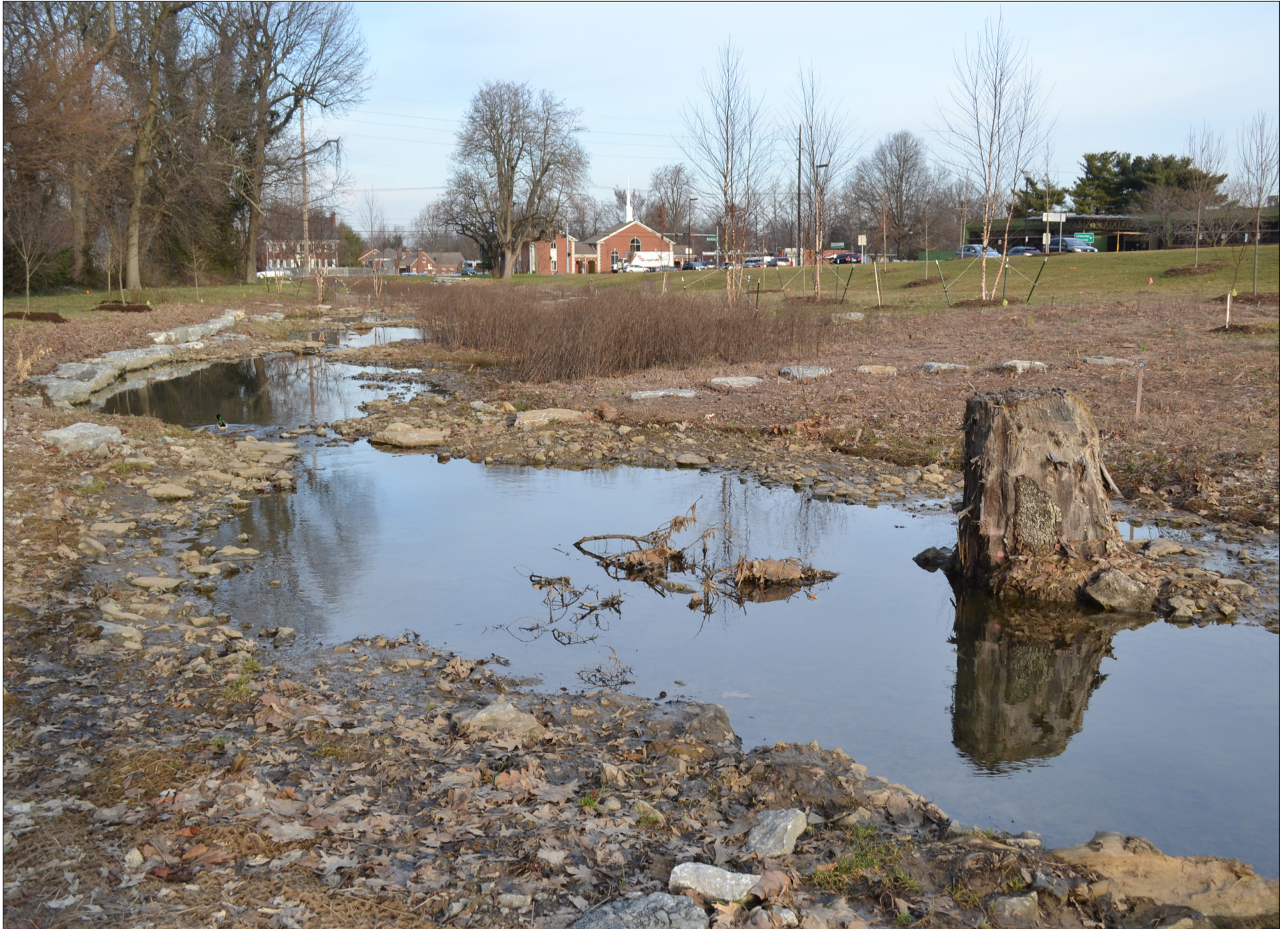
Figure 10. Large-scale stream restoration projects require extensive permitting and specialized engineering expertise.
