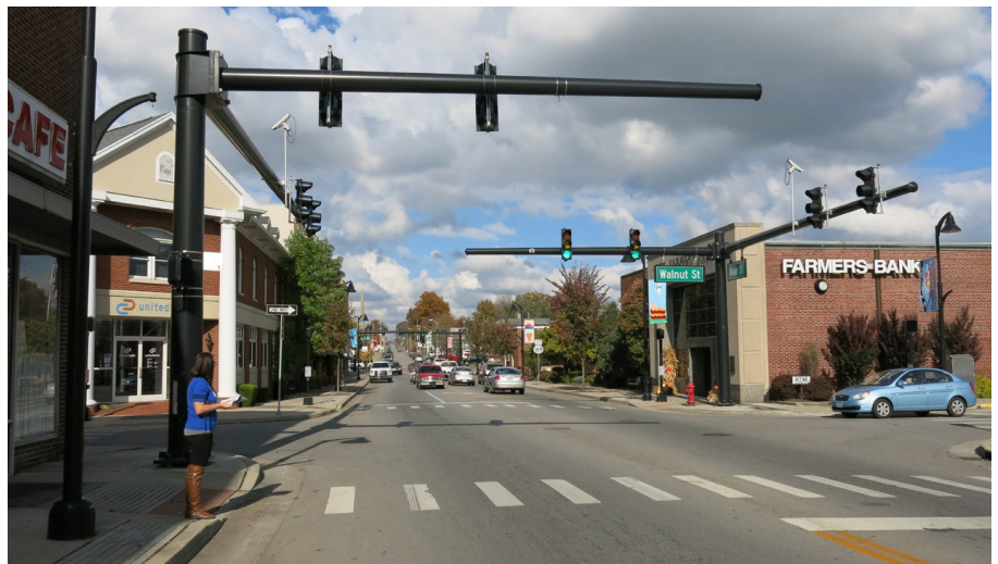
Figure 1. Components of a streetscape. Downtown Owensboro, Kentucky (top), and downtown Nicholasville, Kentucky (bottom)
