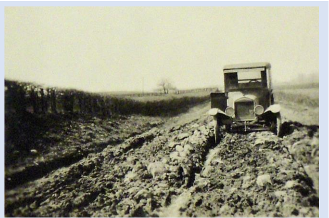
Muddy road near Saint Paris, Ohio, 1921
