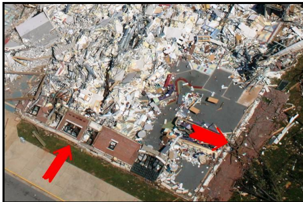
Figure 11. Southeast corner of the Alberta Elementary School. Stacked masonry walls were anchored poorly to the foundation and fell over in the directions indicated (red arrows).
