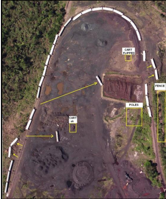
Figure 21. Empty railcars that were blown off the tracks at this coal loading facility.
