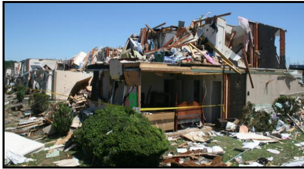
Figure 22. Tornado damage to the Southbrook Apartments in Pratt City. The roof and most second story walls were blown away.
