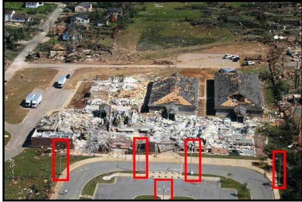
Figure 10. Aerial view of the Alberta Elementary School looking north. Two of the four buildings collapsed. Note the light standards (red boxes) in the parking lot remained upright.
