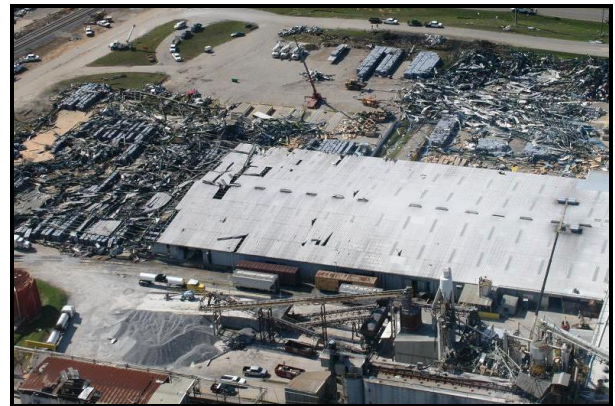
Figure 5. Collapse of metal buildings at the Tamko Roofing Plant.
