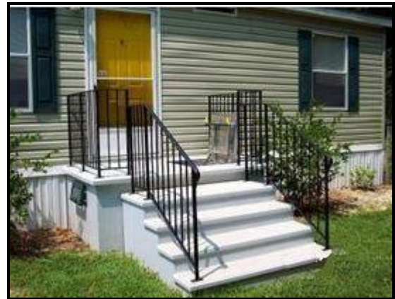
Figure 26. Example of an installed concrete porch shelter with steel entry door.
