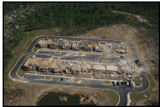
Figure 12. Aerial view of the Chastain Manor Apartments looking north. A portion of the concrete floor slab was exposed on the east end of the south building.
