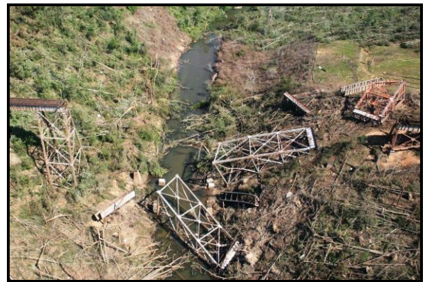
Figure 17. Toppled steel towers that had supported a railroad bridge over Hurricane Creek, northeast of Tuscaloosa.
