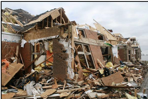
Figure 20. A south facing wood-framed wall on the bank building had been pushed inward, pivoting about its base.
