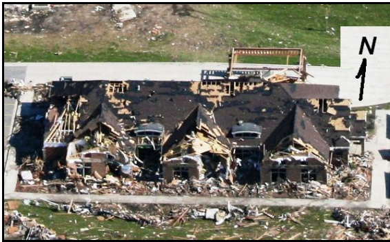
Figure 19. Aerial view of the First State Bank building looking north. The bank was near the center of the tornado path and survived relatively intact.
