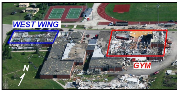
Figure 16. Aerial view of the Parkersburg Community High School looking north. The west wing and gymnasium (outlined) collapsed.
