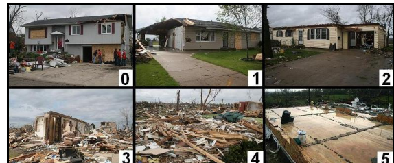
Figure 10. EF-scale ratings to wood-framed houses within the Parkersburg tornado damage path.
