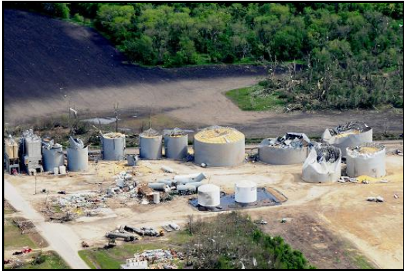
Figure 7. Damage to grain silos filled with corn just east of Parkersburg.
