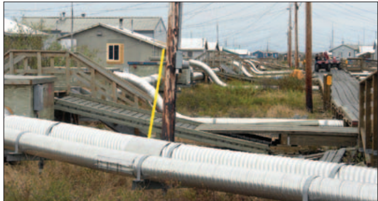
Selawik's streets are a crowded with infrastructure. Mike Brubaker, 2011.
