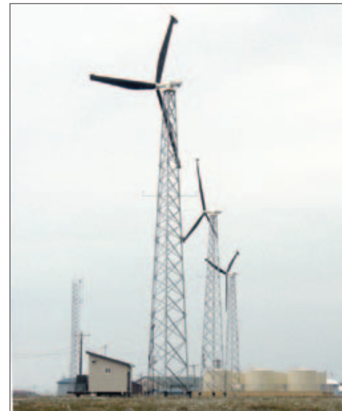
AVEC's 65kw wind generators help power Selawik and control energy costs. Mike Brubaker, 2011.
