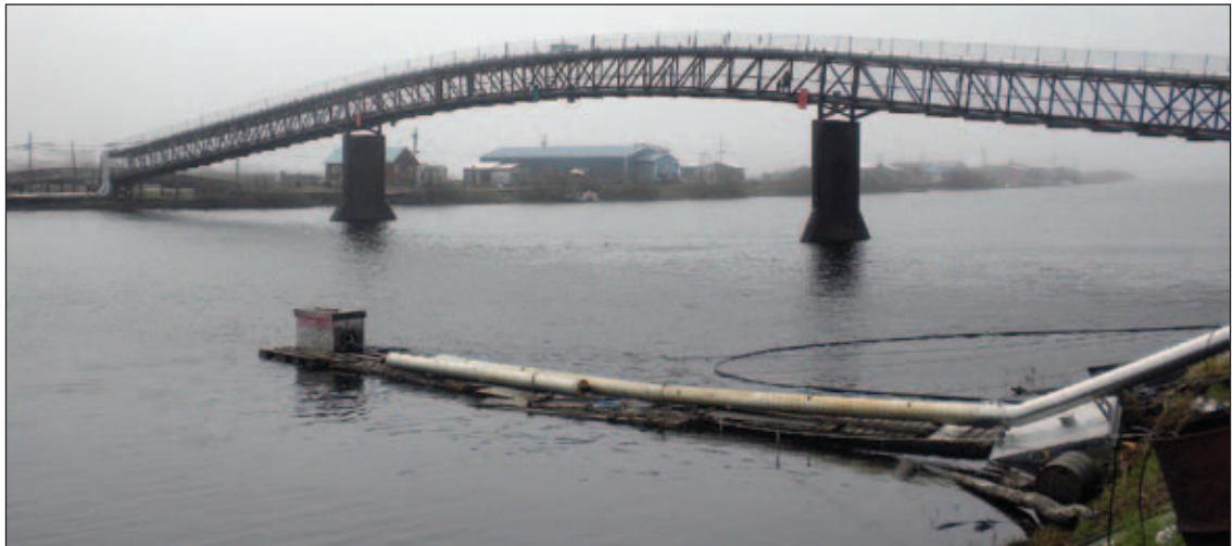
The community water intake. Mike Brubaker, 2011.
