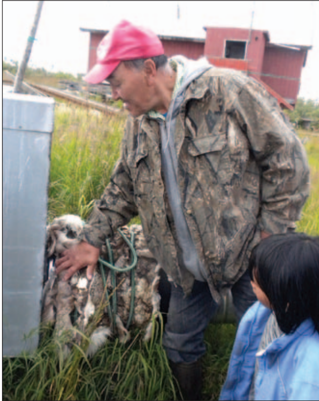
Jackie Snyder used a caribou skin to insulate the broken connection in his Arctic pipe. Mike Brubaker, 2011.
