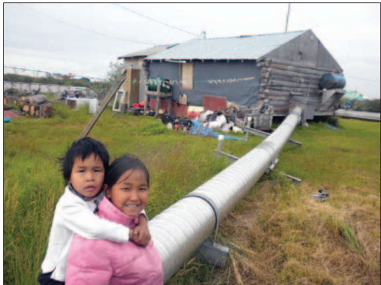
The Snyder kids are all smiles despite the sagging Arctic pipe that brings water to their home. Mike Brubaker, 2011.
