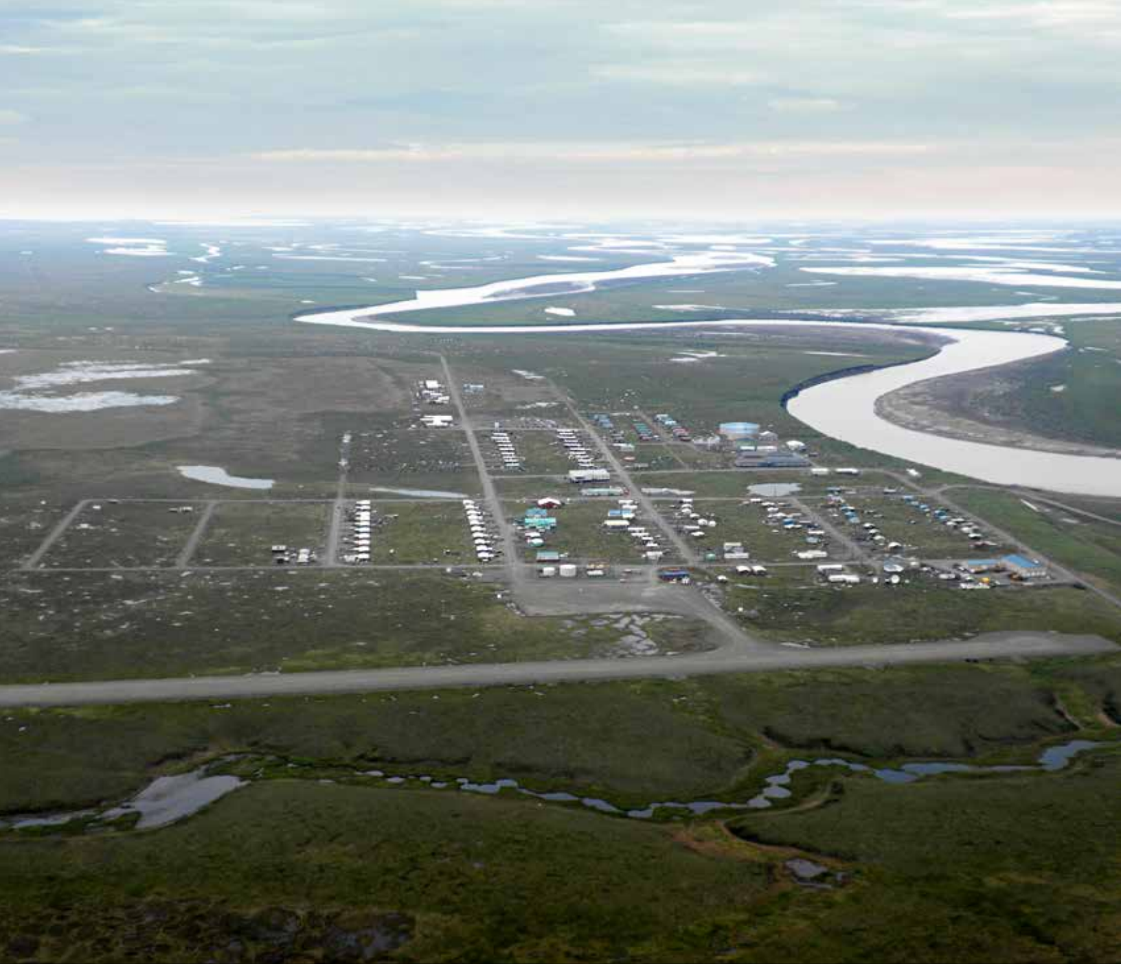
Aerial view of Nuiqsut. Mike Brubaker, 2013.
