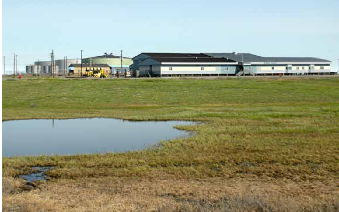
School near eroding river bank. Mike Brubaker, 2013.
