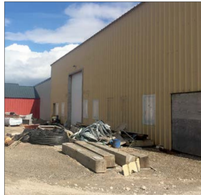
Constructed Meshik Fish Processing Center. Photo by Erica Lujan
