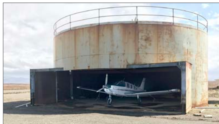
One 250,000 gallon fuel storage tank reused as an airplane hangar. Photo by Mike Brubaker
